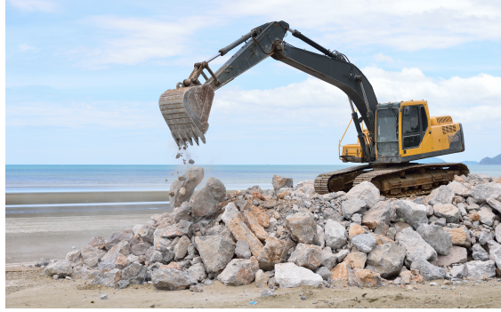
Figure 7.1: Fragmented rocks excavation using an excavator.
